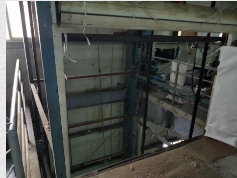
Safety rails removed.....
